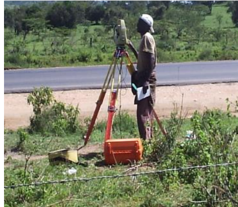
Photo 2: Use of Total Station in road survey.
